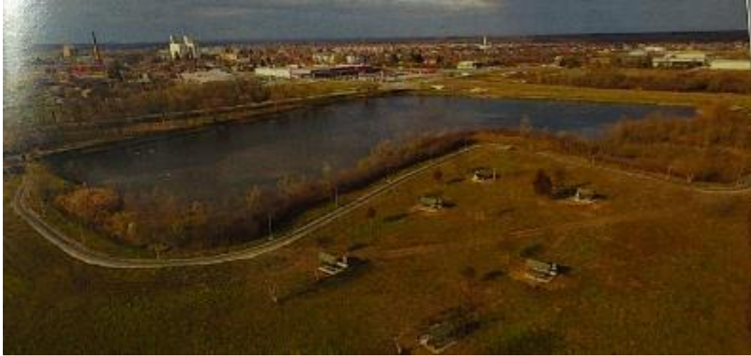
Photo 6. “Brickyard pit” after renovation
